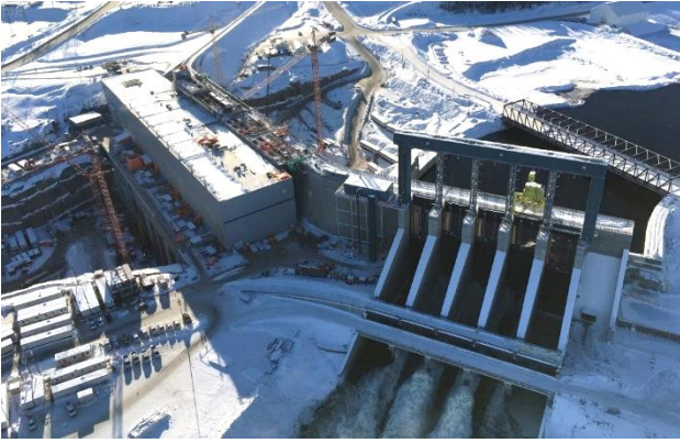
Muskrat Falls Hydroelectric Project – Canada.
